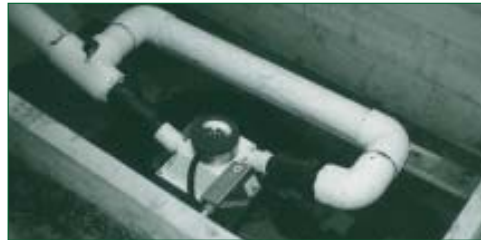
Stream Engine Installation
